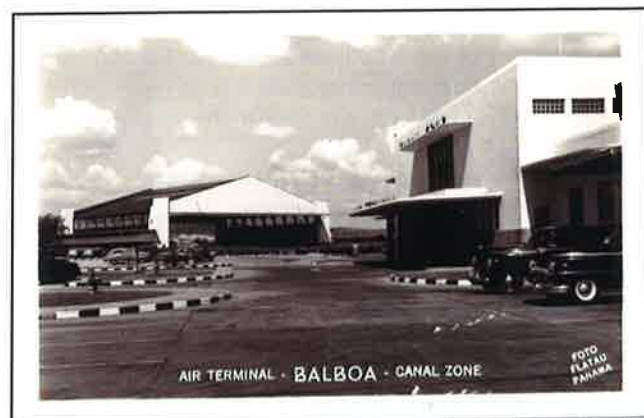
Fig. 3. Balboa Air Terminal -- Showing Hangar.
